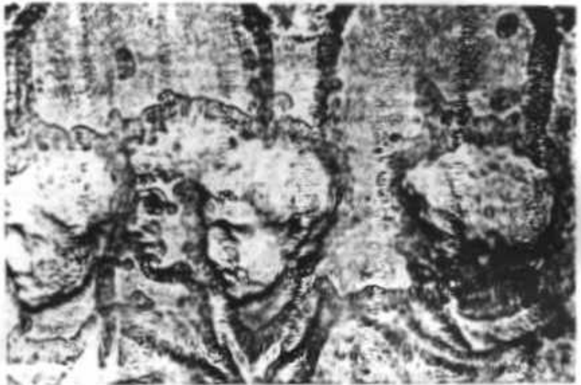
Fig. 1. Details of relief on Trajan's Column (in 1959) where the isolated pits are prominent on vertical parts and long depressions caused by joined pits or induced in a different way are common throughout.
