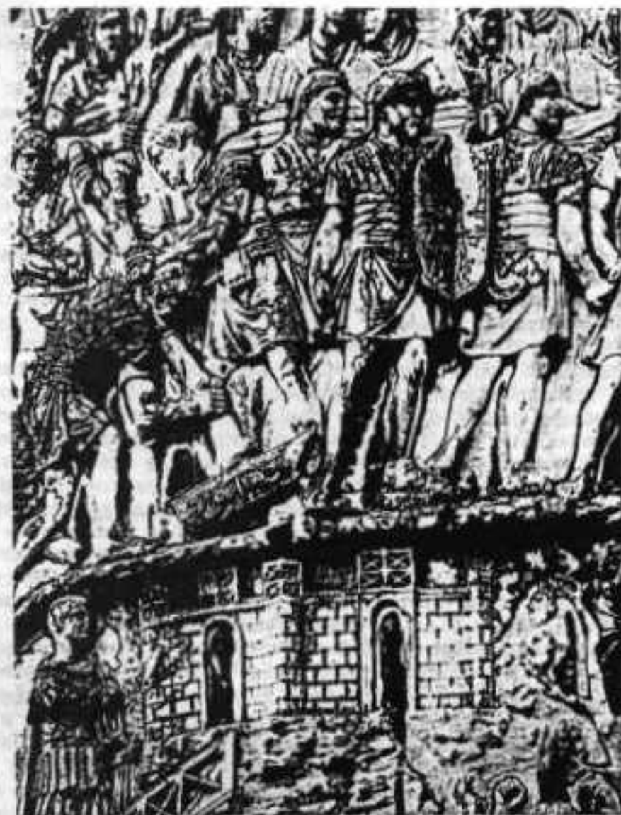
Fig. 3. Trajan's Column at the end of the 19th Century. Dark crust, possibly of cyanobacteria, is prominent in long and circular depressions. Such a crust does not exist there at present (cf. Fig. 1).
